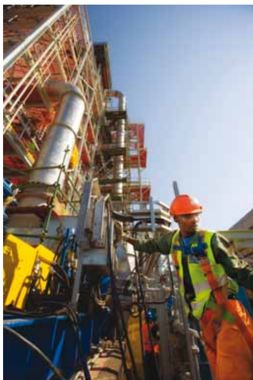
Construction of the new RBMR tankhouse
