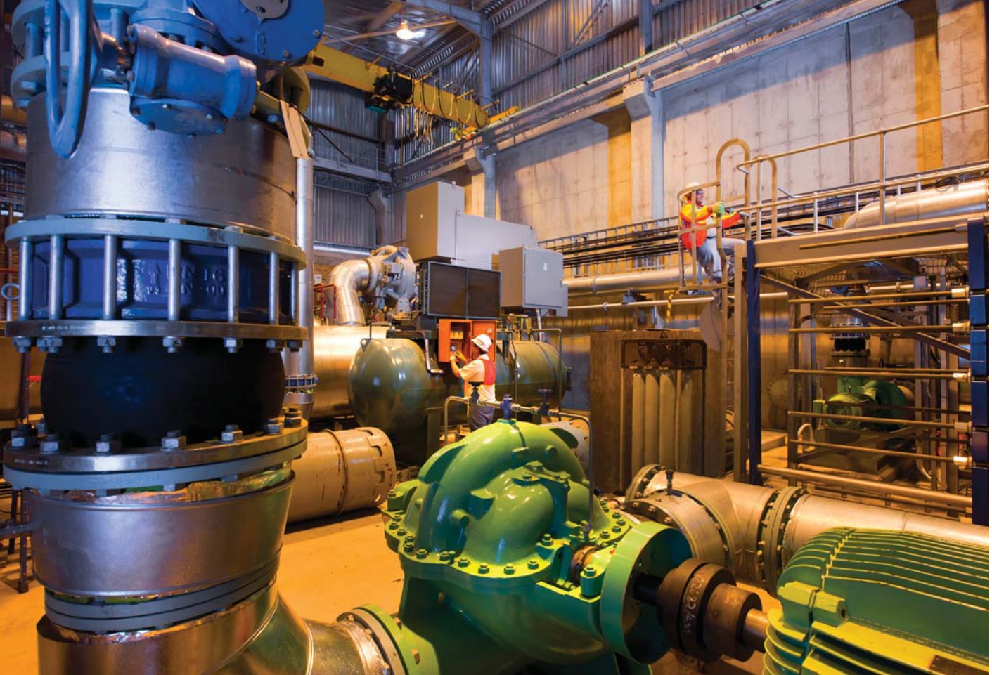
New refrigeration plant at Anglo Platinum Limited's Khuseleka Mine.
